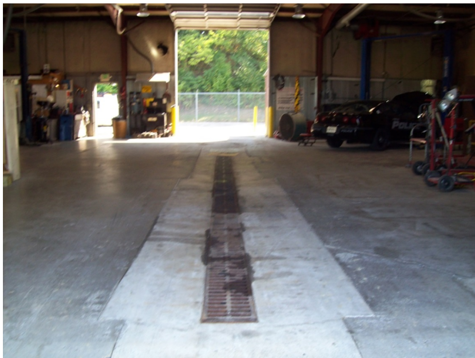
Service Bay Grate Drain that is Connected to Sanitary Sewer with Separator – July 2015
