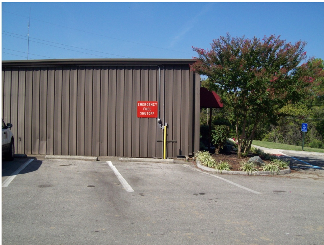
Emergency Fuel Shutoff Across the Fueling Station – July 2015
