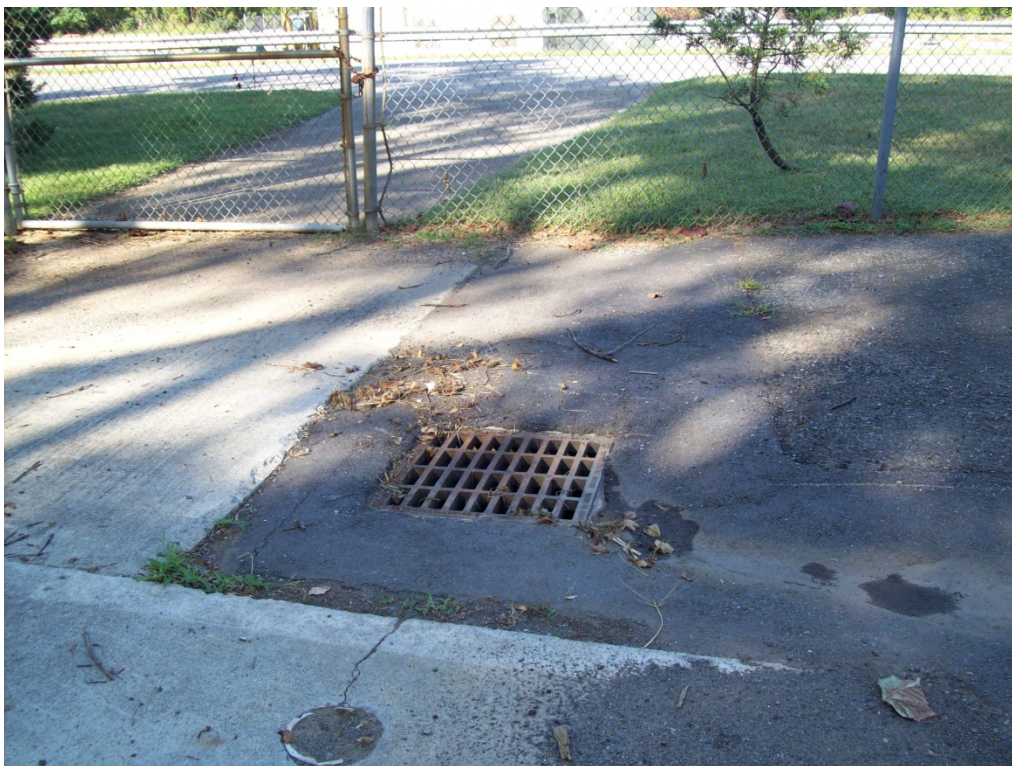
Drainage Inlet in the Town Vehicle Parking Areas with Separator – July 2015
