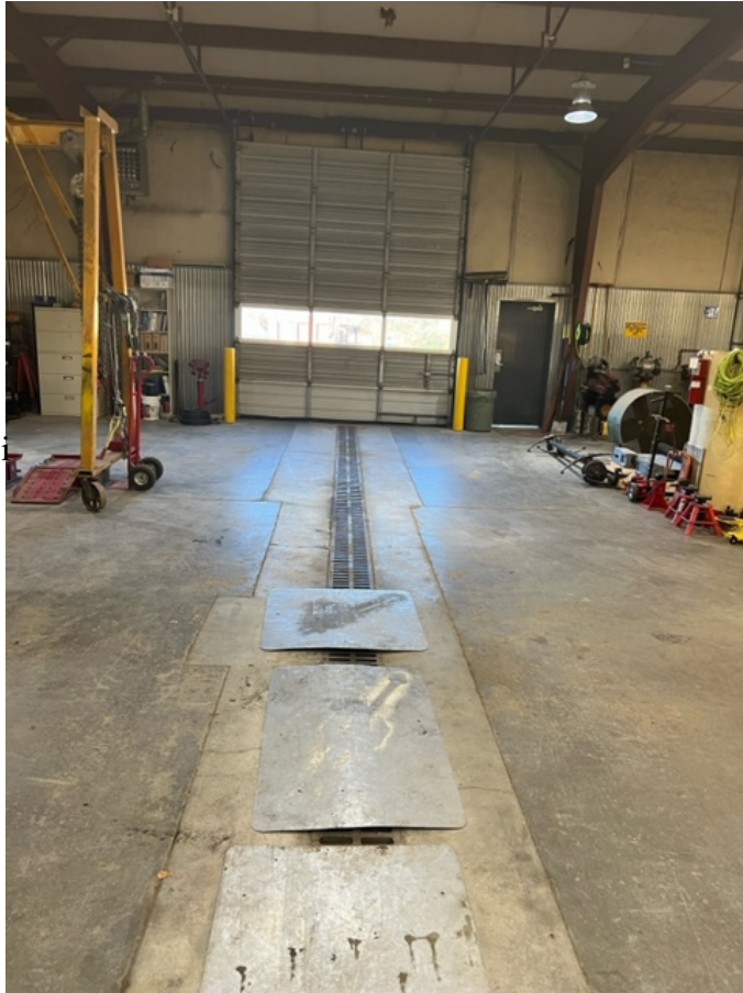
Service Bay Grate Drain that is Connected to Sanitary Sewer with Separator – November 2022
