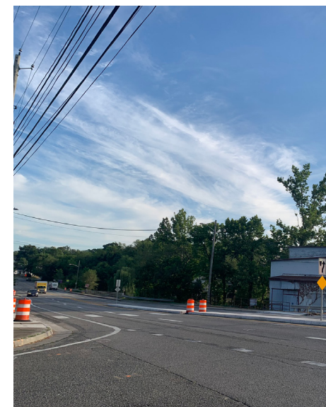
Crosswalk under construction at Gish Mill
