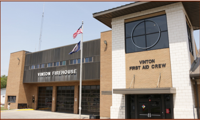
Vinton Fire and Rescue Station 2
